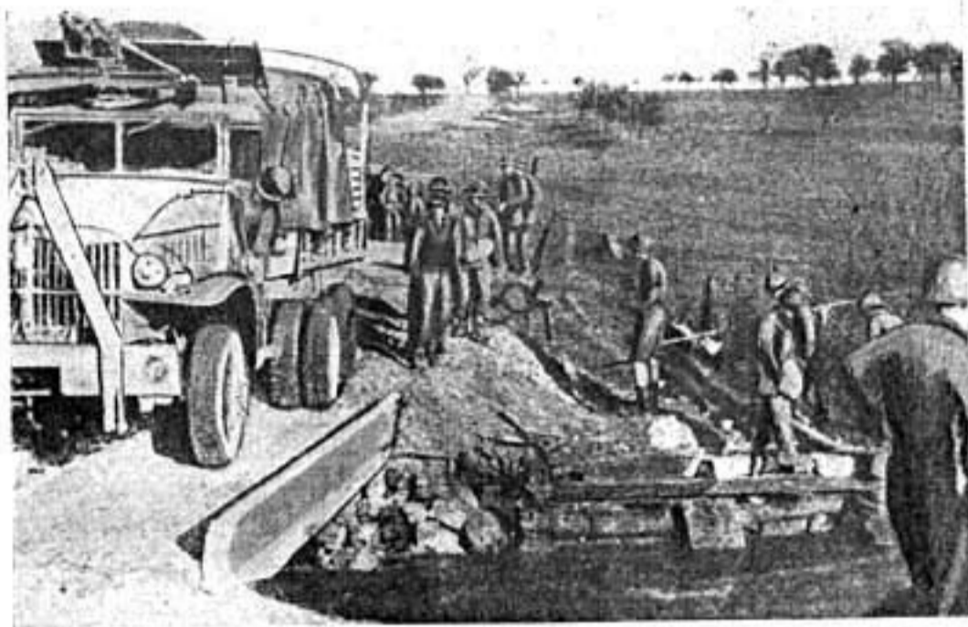
The Bridge at Nieffern
